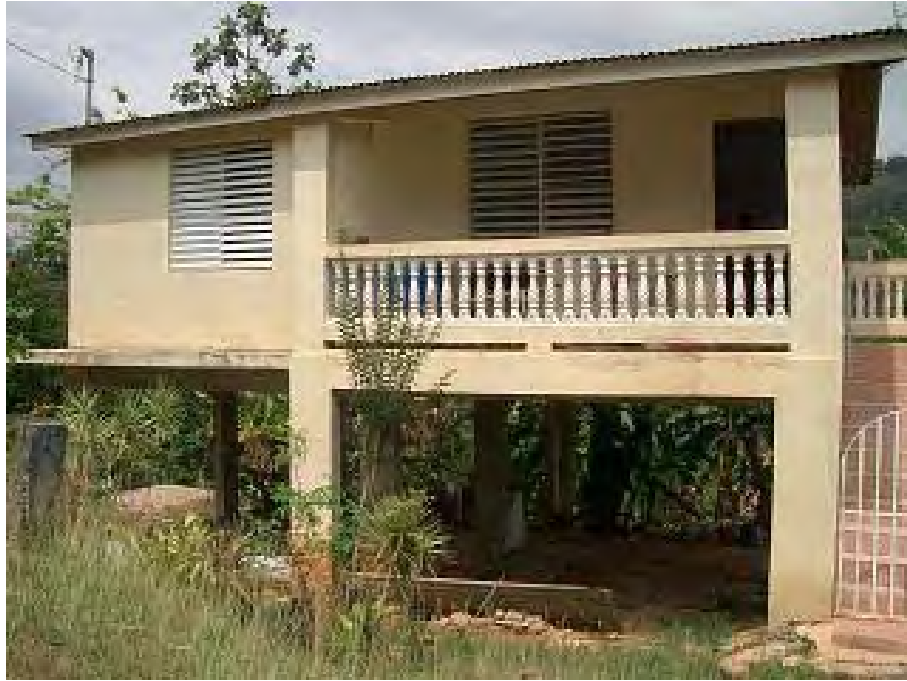
Figure 4-5 House with gravity columns
